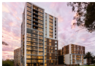
Highline, Westmead 556 apartments
