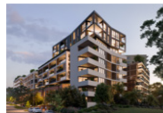
Proximity, Rouse Hill 375 apartments
