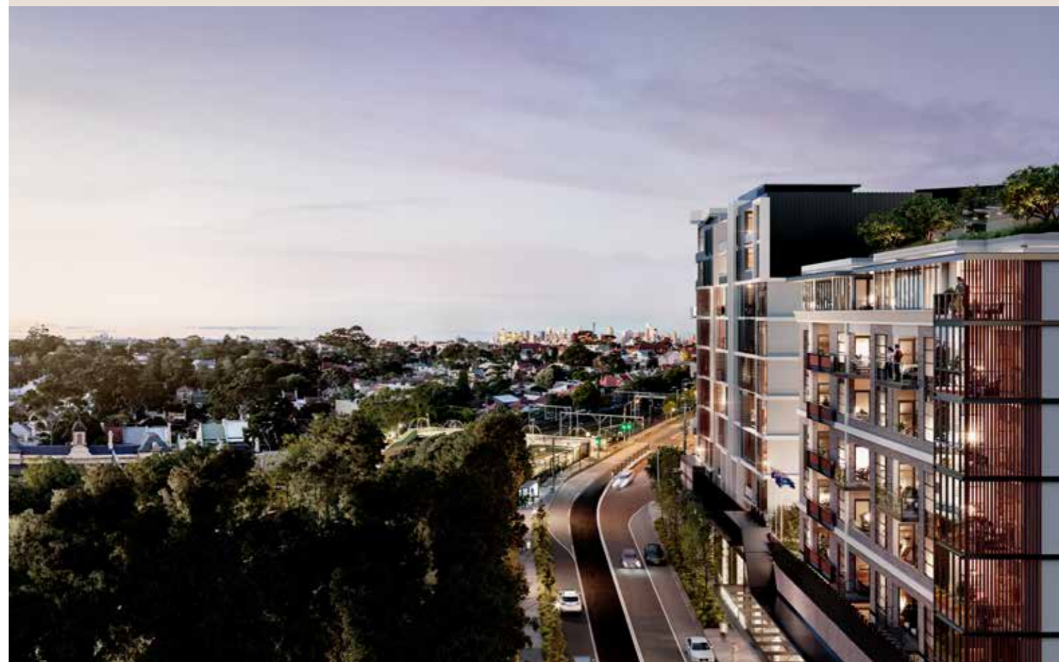
The Siding, Petersham - Under Construction
