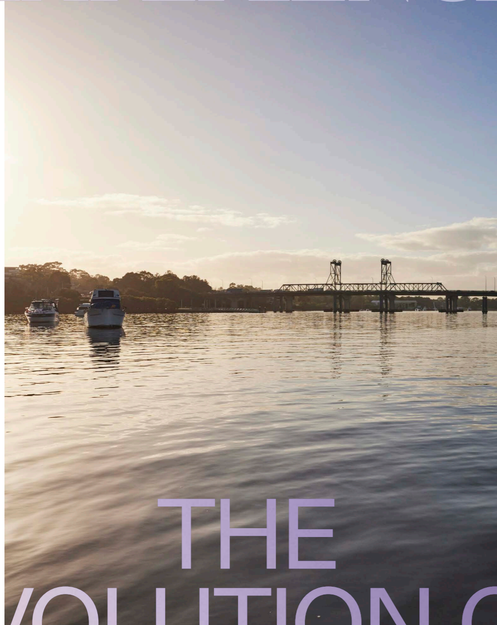
VIEW OF RYDE BRIDGE
