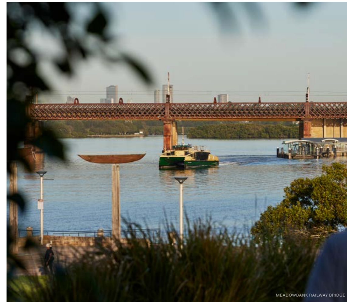
MEADOWBANK RAILWAY BRIDGE
