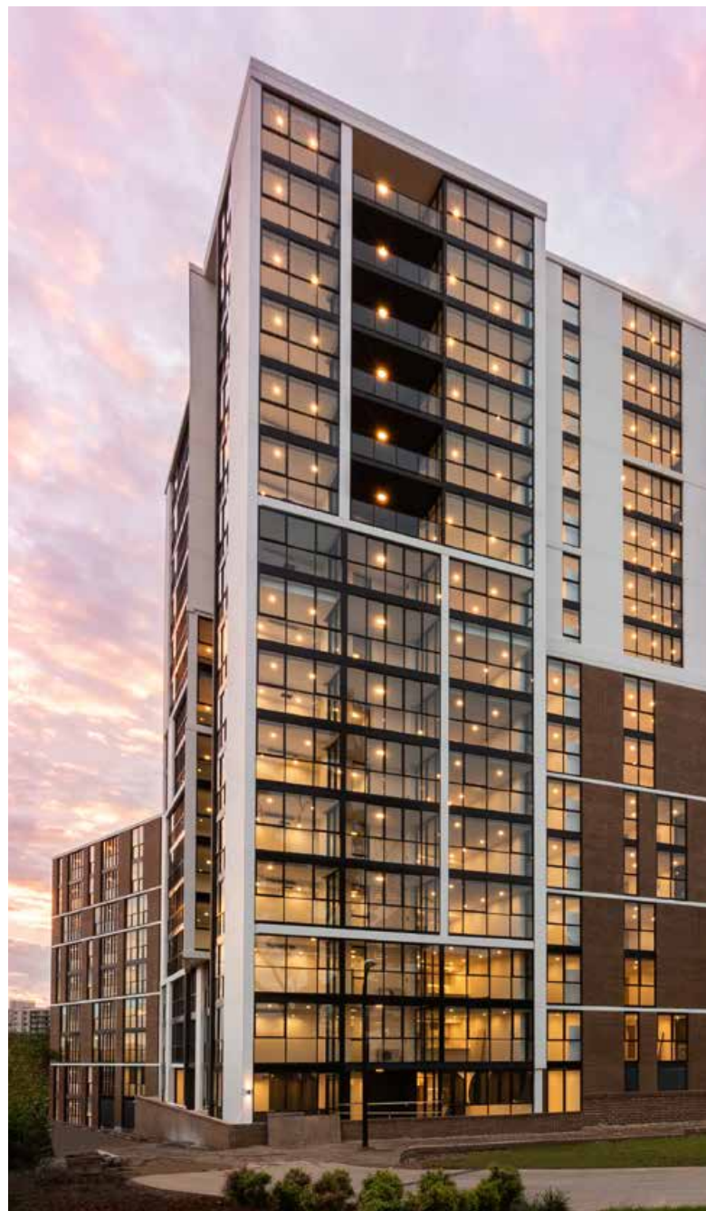
HIGHLINE, WESTMEAD 555 apartments
