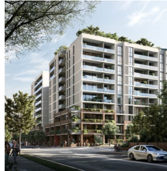
TIAN AN LFD Developer
